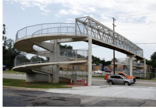
(b) Truss Bridge
